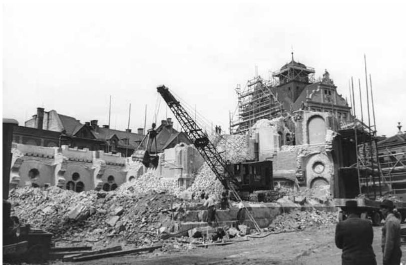
Abbruch der Münchner Hauptsynagoge, Juni 1938 Demolition of Munich's Main Synagogue, June 1938
